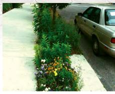
Stormwater planters in Philadelphia capture and filter stormwater runoff from an adjacent roadway.
