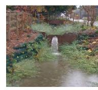
A stair-stepped pool slows runoff in Seattle's NW 110<sup>th</sup> Cascade project.
