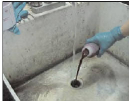
Figure 63: Dye Testing Plumbing (NIWPC, 2003)
