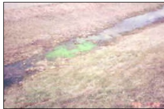
Figure 73: Dye surfacing in a septic field
