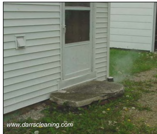
Figure 71: Smoke Rising from Sewer Vent
