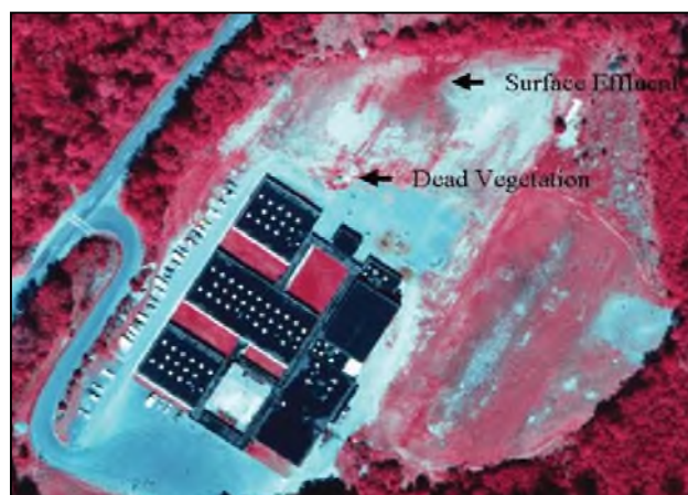
Figure 75: Dead vegetation and surface effluent are evidence of a septic system surface failure. (Source: U.S. EPA, 1999)
